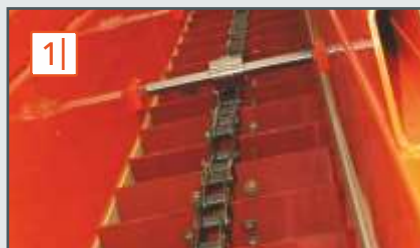
1| New elevator guides.
