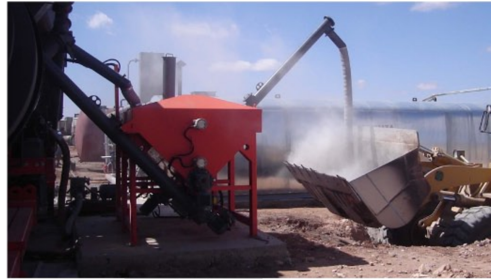
Unloading of excess fine aggregates
